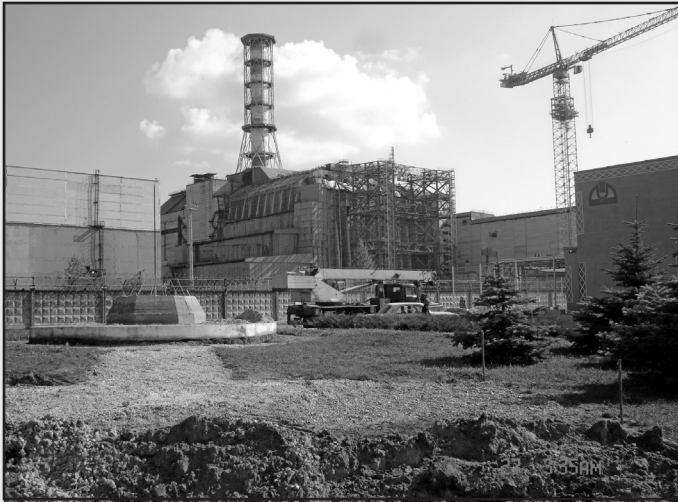
Figure 4: The sarcophagus which covers the remains of the reactor, taken from the back of the view in Figure 2.
