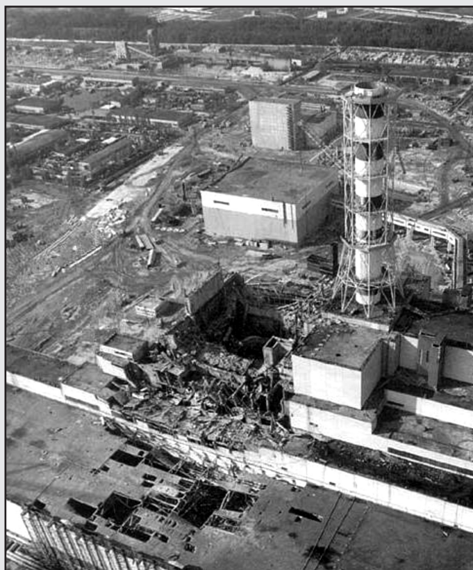
Figure 2: Chernobyl Reactor #4 - This is probably taken from a helicopter several days after the explosion. The reactor was in the center of the photo and apparently has stopped burning. The photographer is unknown. It is published under the fair use rationale.
